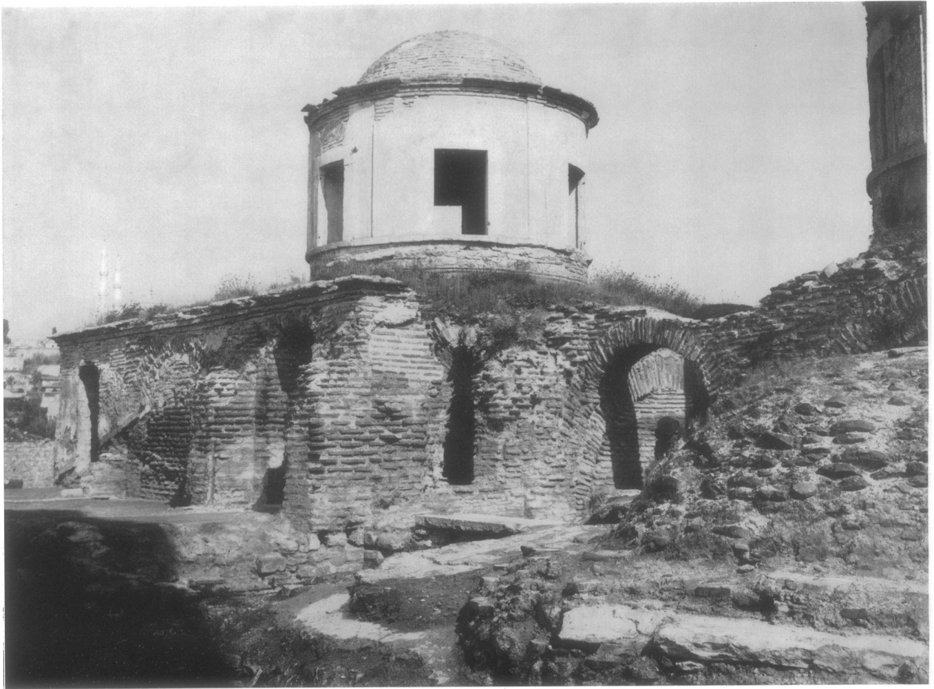
12. Superstructure from Southwest
