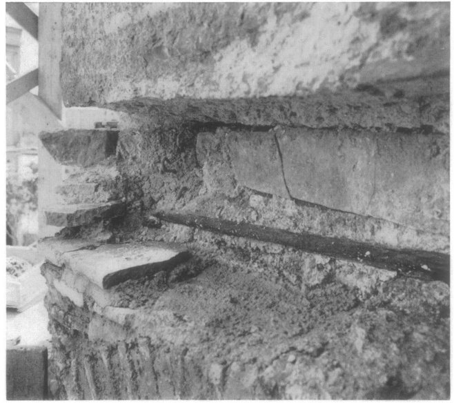
9. Fenari Isa Camii, Main Apse, Wrought Iron Collar below Inscribed Cornice
