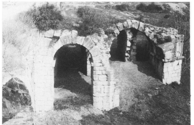
(e) First phase vaults from west.
