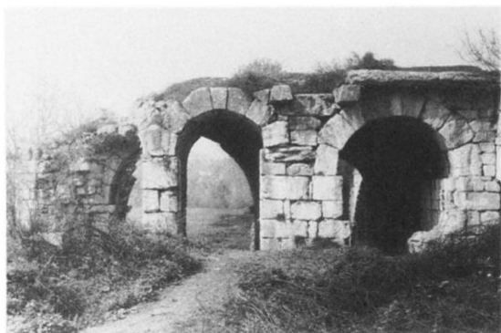
(c) Second phase vaults from east.
