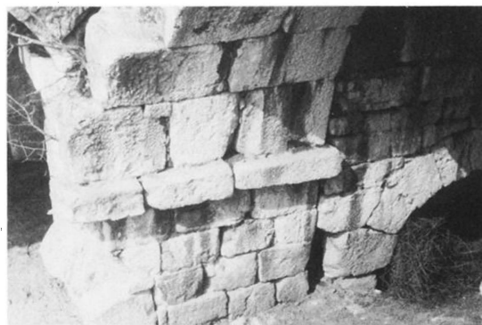
(d) Middle pier of vaulting, showing join of first phase (with cornice) and second phase (with water channel).
