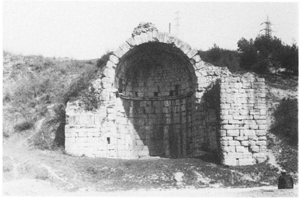
(c) Apse at east end of bridge.
