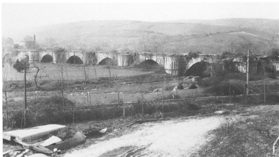
(b) South side of bridge looking west.
