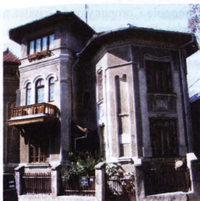
The first house subject to allotment, at the crossing between Clucerului and Ady Endre
