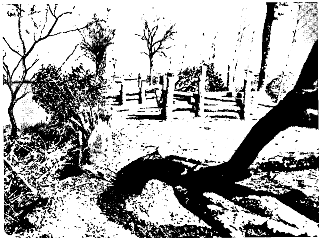
Figure 24. A log obstacle constructed by engineers.
