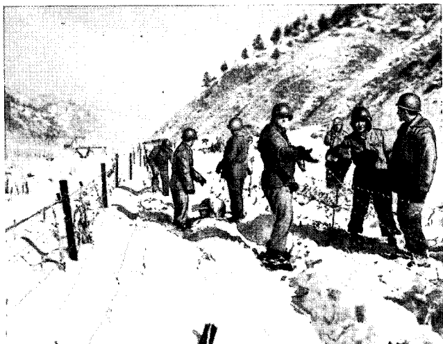
Figure 9. Engineers constructing a barbed wire fence.
