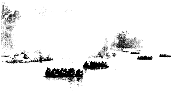
Figure 17. River-crossing operations, assault phase.
