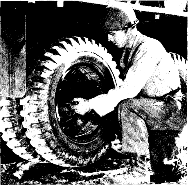
Figure 53. Substitute for a jack to remove outside dual wheel.
