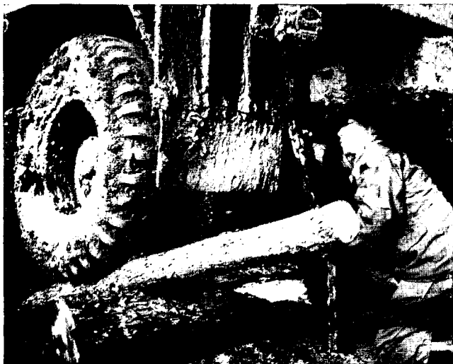
Figure 57. Raising tandem axle.
