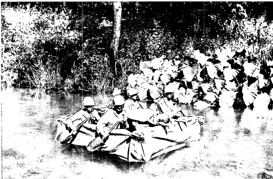
Figure 232. Litter and paulin raft, construction.
