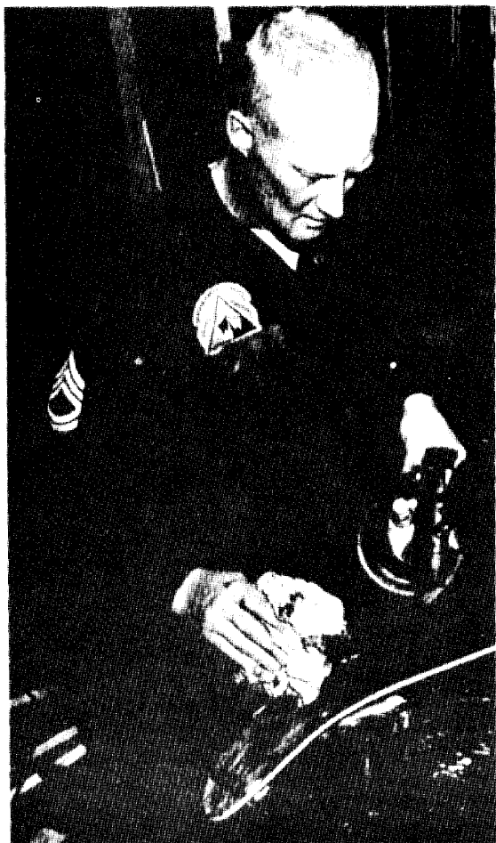
Figure 4-5. Heating pine tar with a blowtorch.
