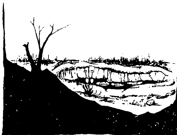
Figure D-1. Emplacement after excavation of all loose earth.
