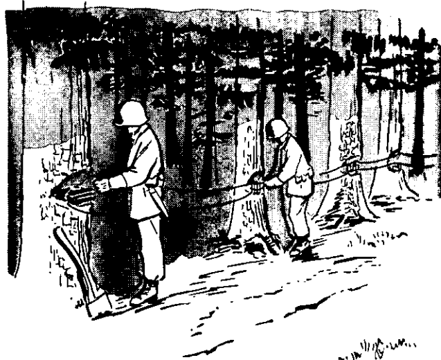
Figure 7-9. Preparing explosive charges for abatis construction.
