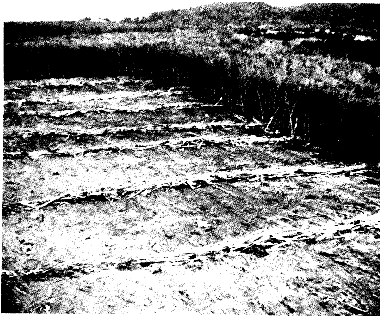
Figure 3-34. Clean, well compacted windrows prepared for burning.
