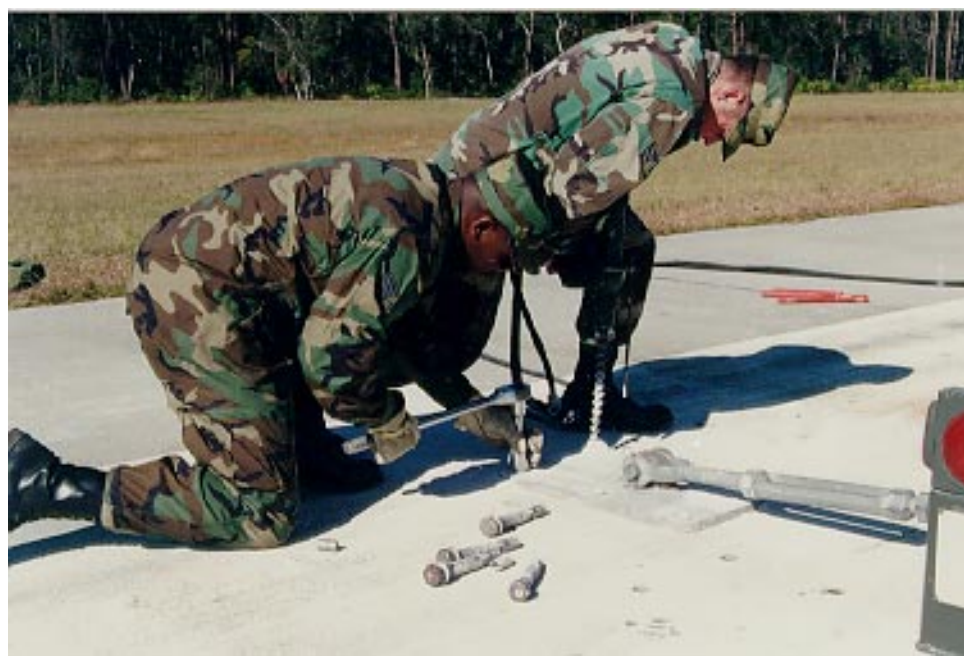
Figure 8.11. Anchor Plate Installation.
