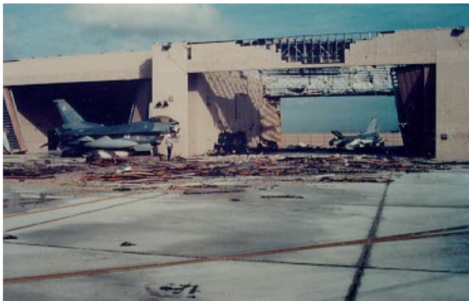
Figure 6.1. Air Base Facility Damage.
