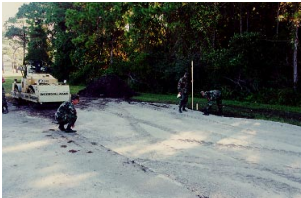
Figure 11.5. Alternate Route Under Construction.
