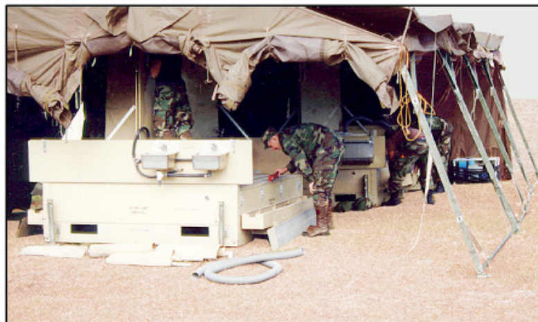
Figure 22. Installing a Field Deployable Latrine.
