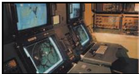
Fire Distribution Center
