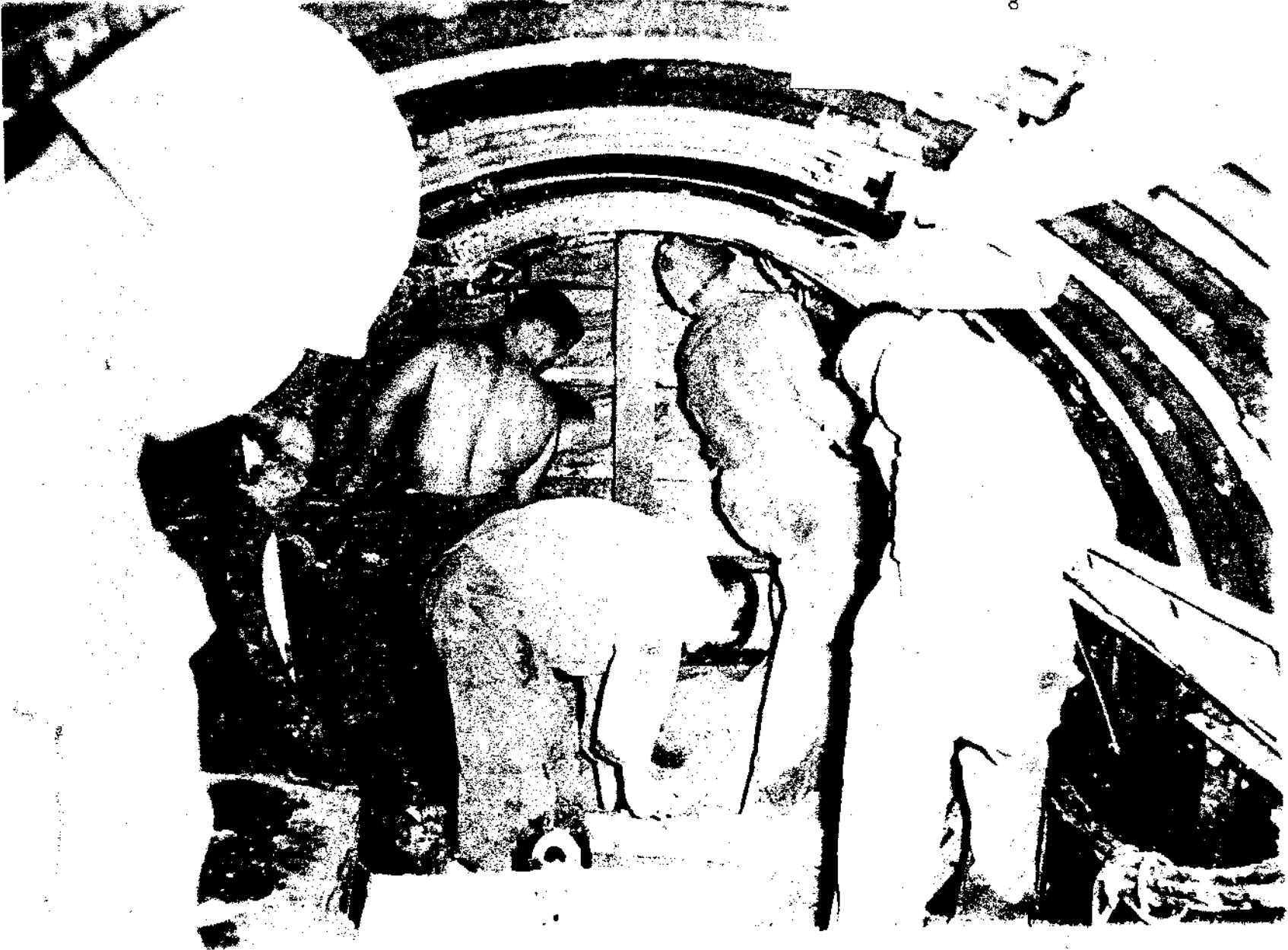
Figure 8 - Excavating Using the Blinds
