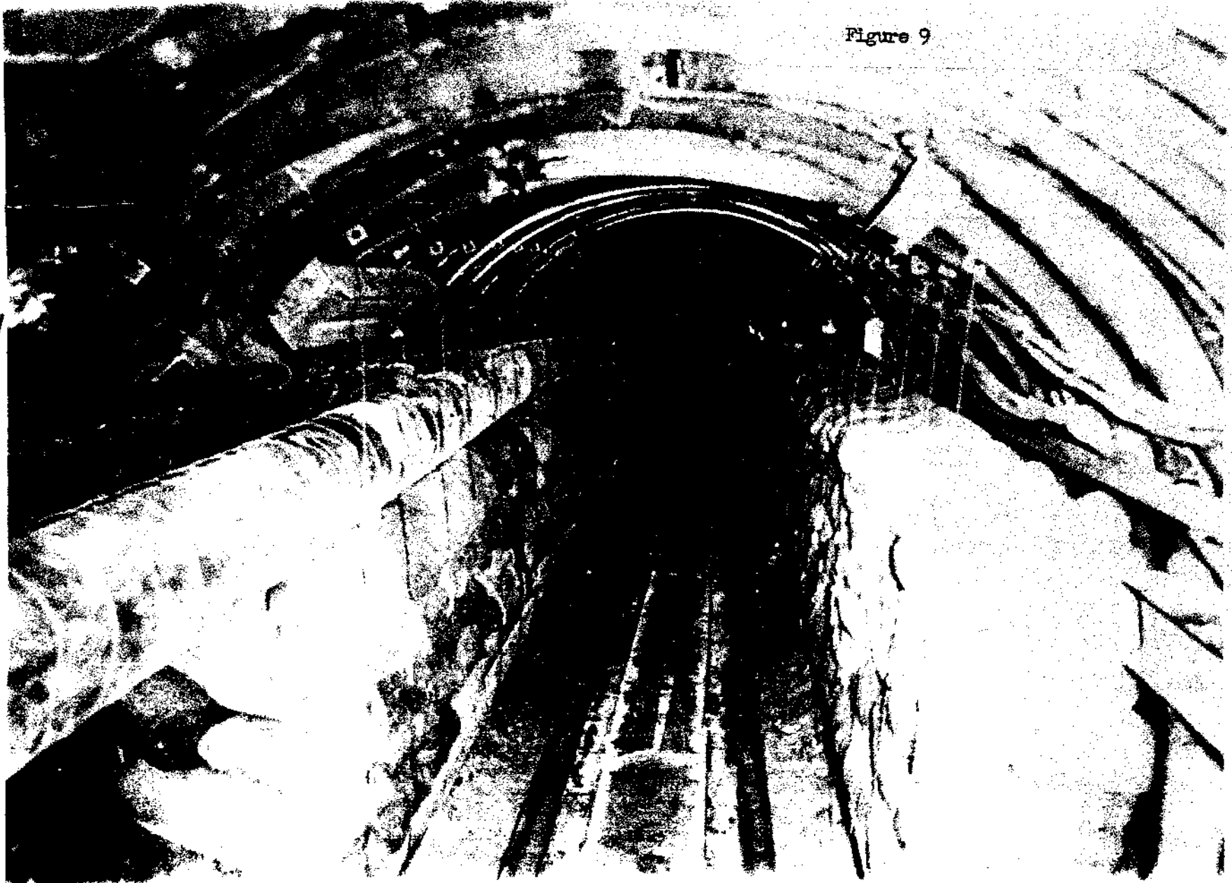
Figure 9 - View of the Completed Tunnel
