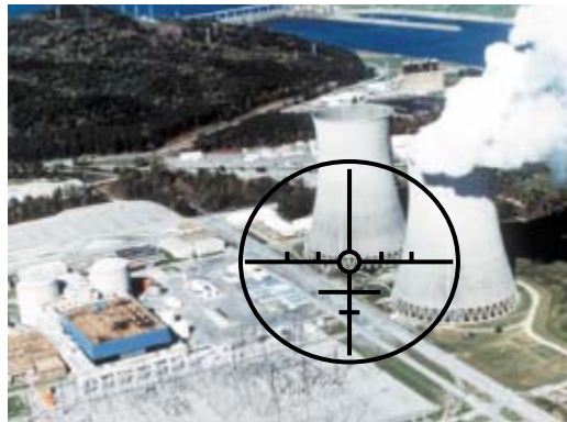
Figure. I-1. Nuclear Plant Photo
