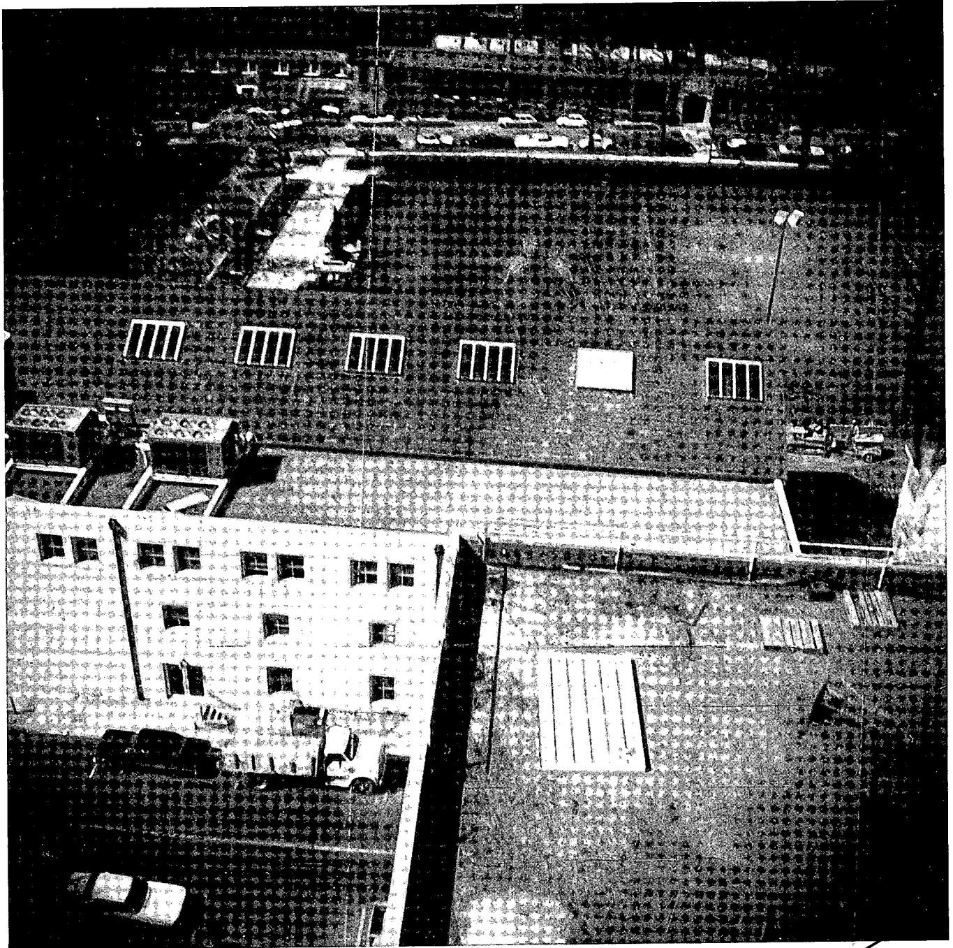
FIGURE 22. Roof Top with Air-Conditioner
