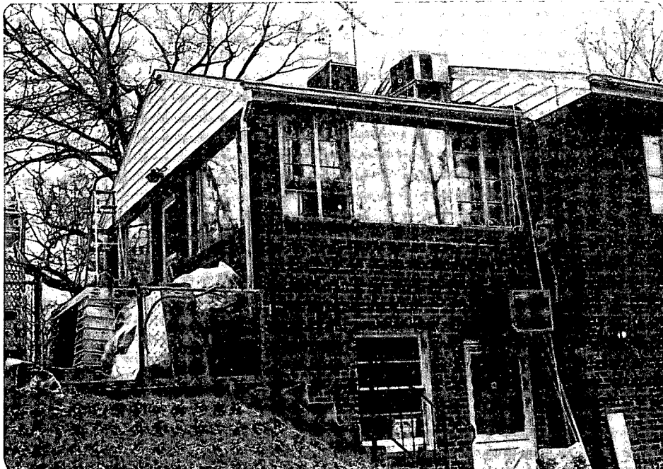
FIGURE 34. Exterior View of the Attic Loft
