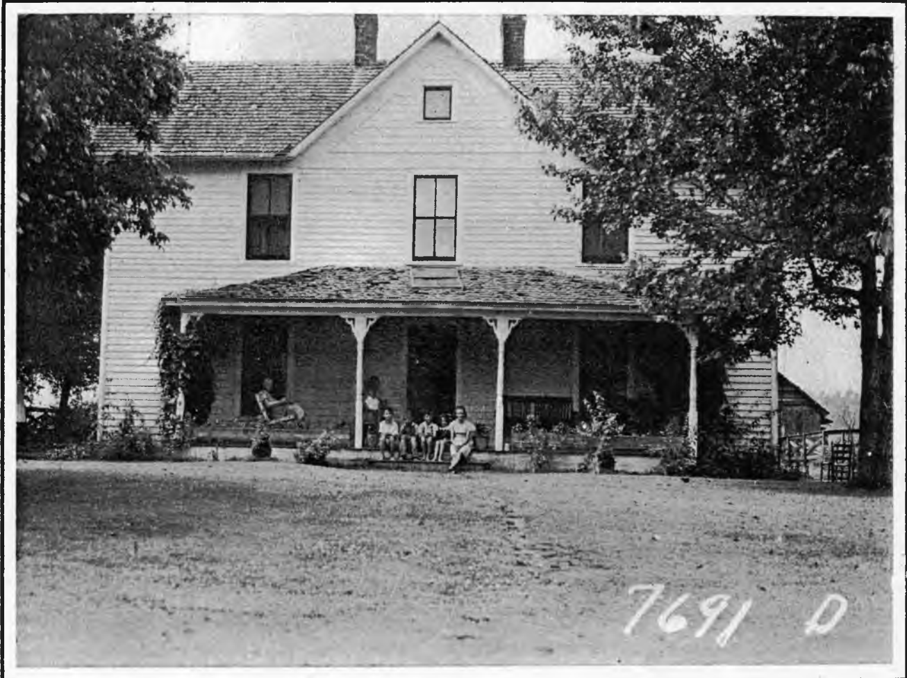
OWNER-OCCUPIED FARM RESIDENCE - ROANE COUNTY
