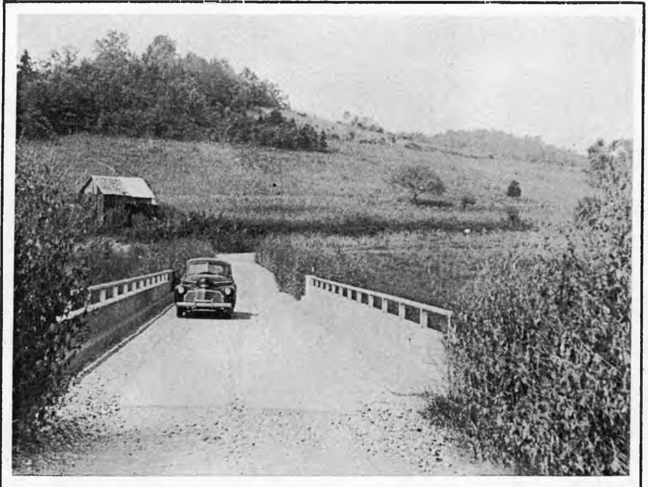
EAST FORK BRIDGE - MCKINNEY ROAD
