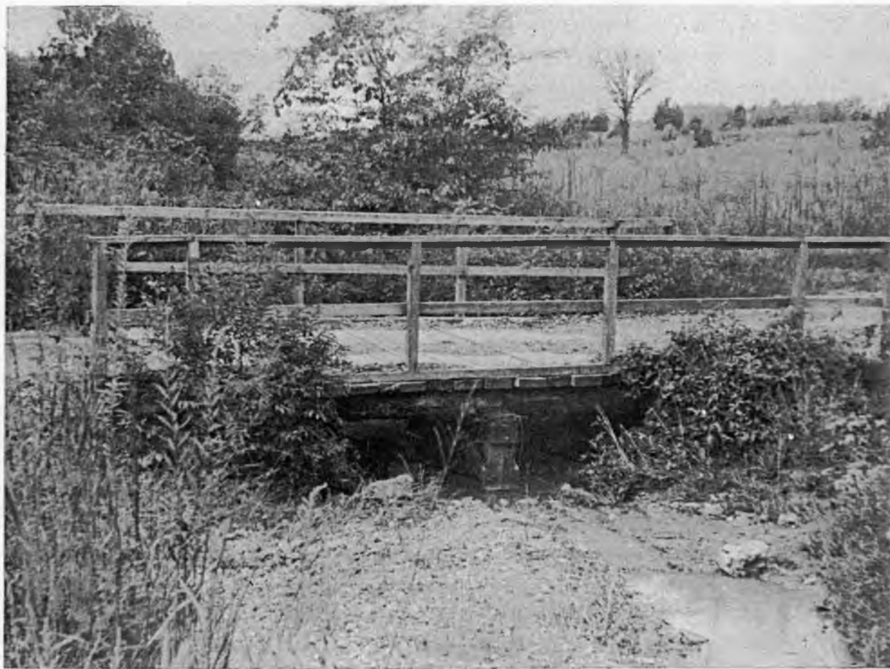
WOOD BRIDGE OVER GRASSY CREEK
