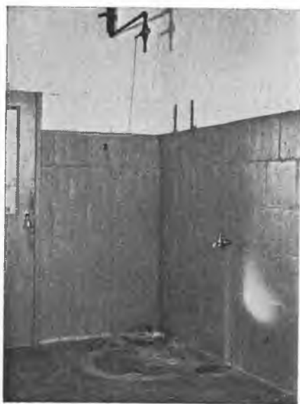
Courtesy Hercules Powder Company Figure 5. Emergency shower bath provided with quick-opening valve for quickly flushing chemicals from the clothes or body. Other types have a platform-actuated valve. (See paragraph 39.)
