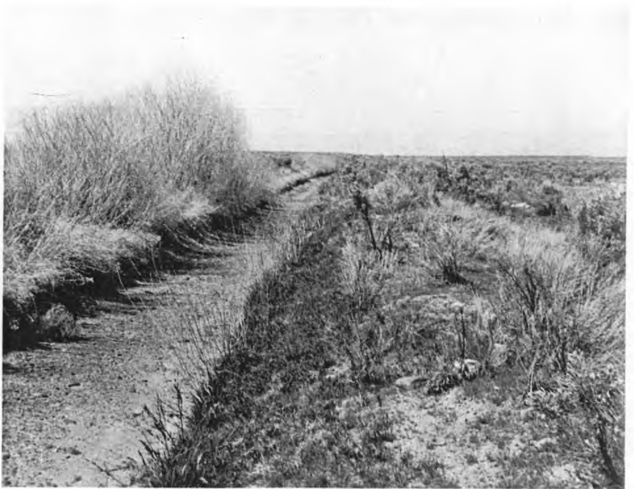
Typical Irrigation Ditch serving the Priest Rapids Irrigation District, in the Hanford-White Bluffs area. This section of ditch is about 1\frac{1}{2} miles southwest of White Bluffs.
