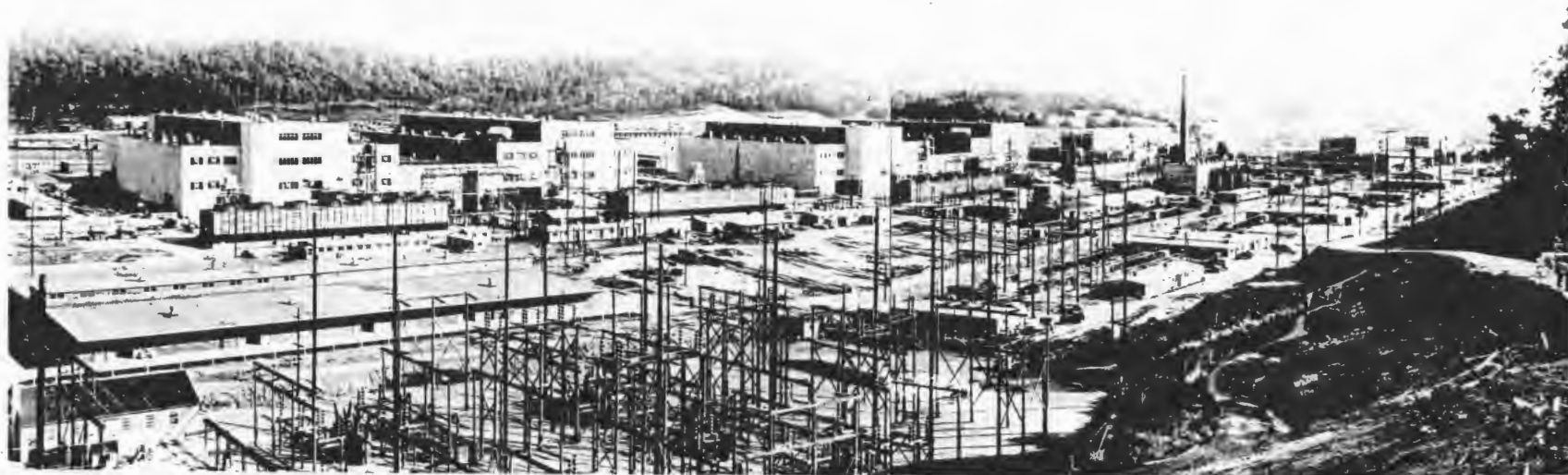
Y-12 EXTENSION AREA VIEWED FROM SOUTH, JANUARY 1945. MAIN PROCESS BUILDINGS IN CENTER.
