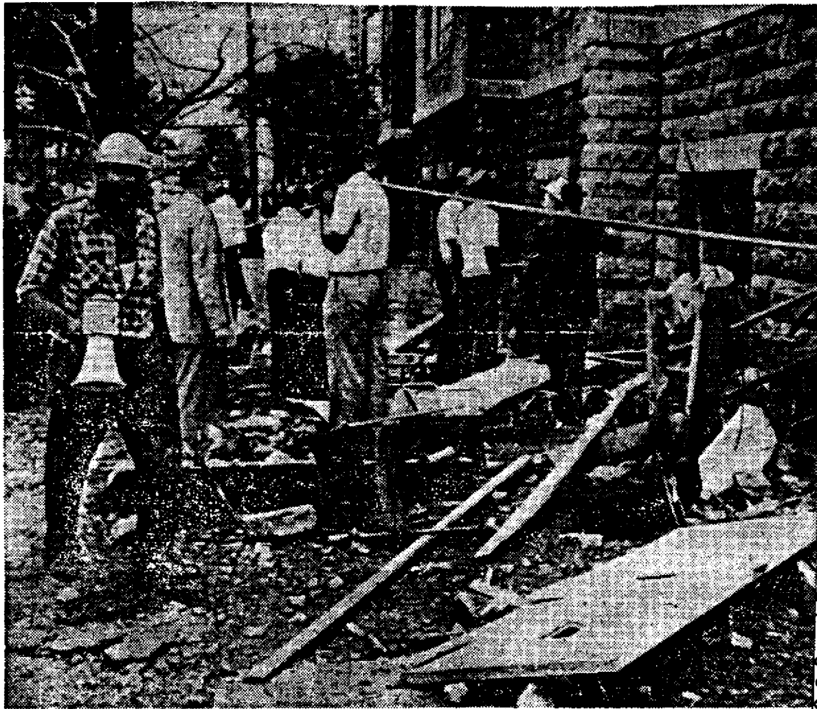
A Civil Defense worker in the foreground carries a bull horn as he and firemen inspect the debris from the bombing of a church
