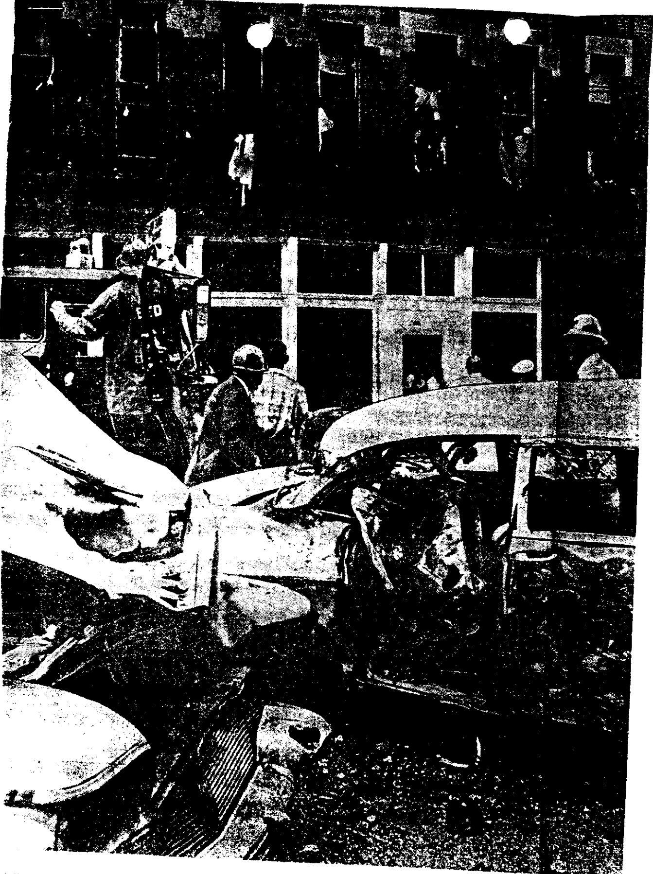
SHROOMING EXPLOSION SHATTERED CARS, STRUCK BUILDINGS News Staff photo—Tom Self Photograph shows damage caused across street from church
