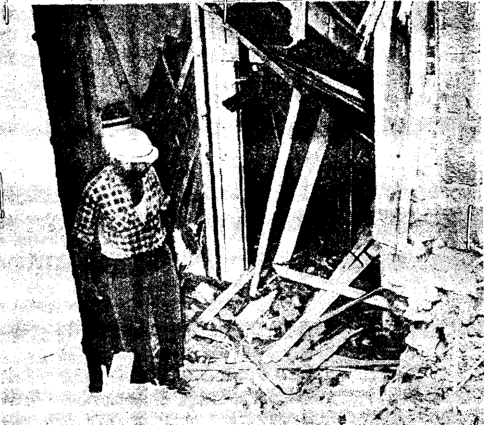
WHERE BOMB WENT OFF —A law enforcement officer inspects the broken timbers and debris in the rubble of the Sixteenth Street Baptist Church, where a dynamite bomb killed four persons yesterday. The bomb ripped out the wall of the building, as shown above, and scattered glass and wreckage into the street.
