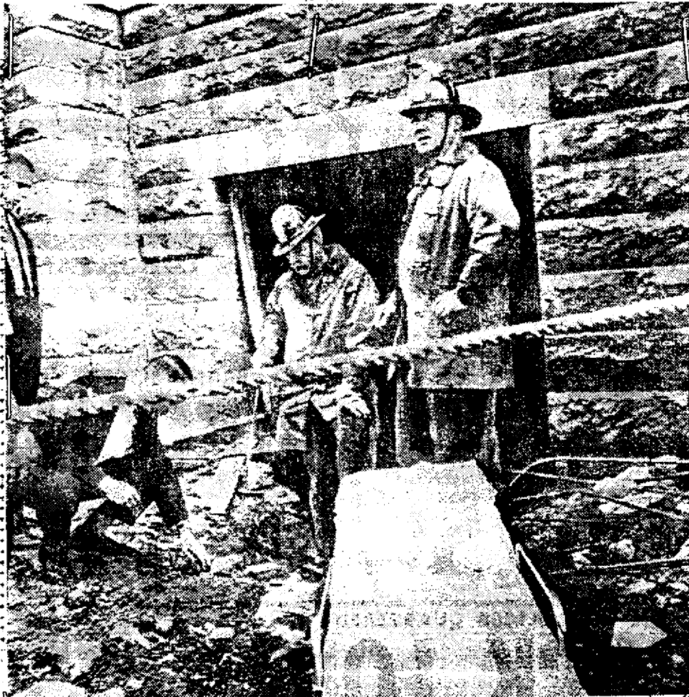
FOR VICTIM —Birmingham firemen and policemen helped ambulance personnel clear the way through the debris of the bombed-out Sixteenth Street Baptist Church yesterday, in an effort to bring victims and survivors out of the rubble. Four persons were killed and more than a score injured in the blast.
