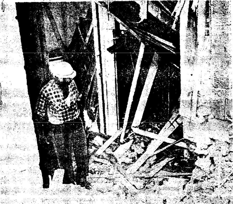
WHERE BOMB WENT OFF —A law enforcement officer inspects the broken timbers and debris in the rubble of the Sixteenth Street Baptist Church, where a dynamite bomb killed four persons yesterday. The bomb ripped out the wall of the building, as shown above, and scattered glass and wreckage into the street.
