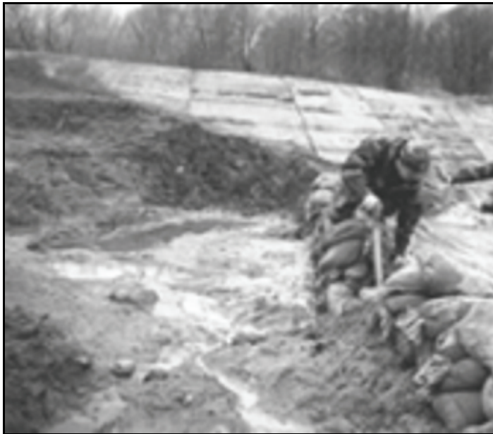
Figure 6-2. Digging a dike/berm.
