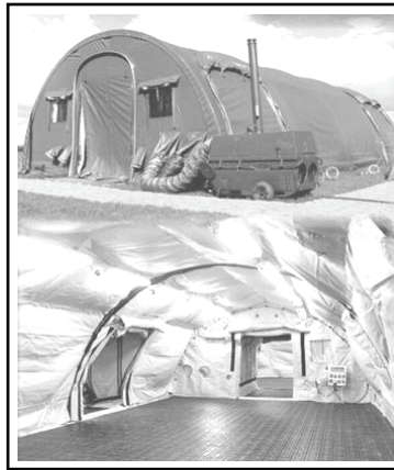
Figure 10-6. Rubb fabric structure
