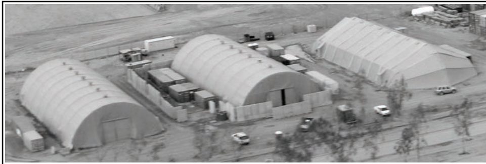
Figure 10-7. Tension fabric structures located at Balad Air Base, Iraq
