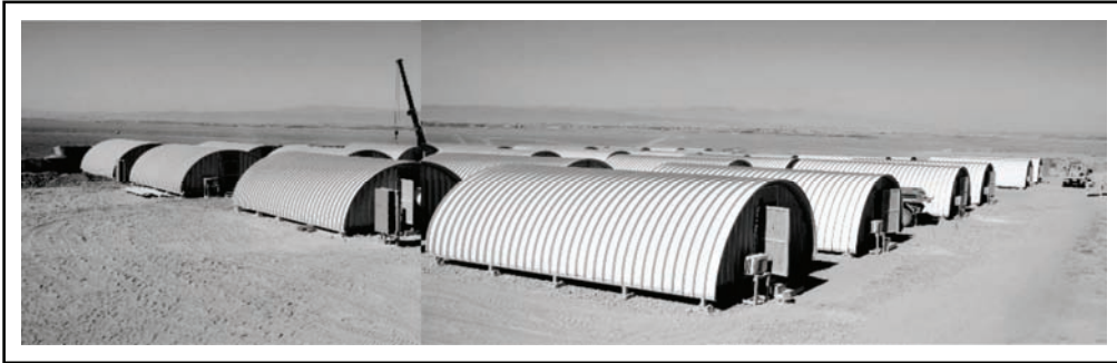
Figure 10-4. Metal buildings constructed with the UBM in a contingency environment
