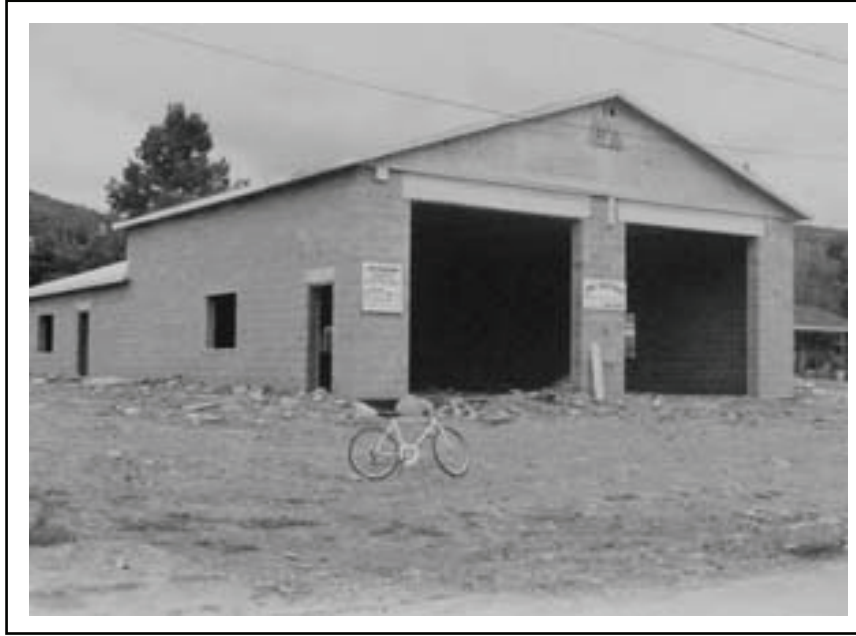
Figure 10-11. CMU constructed fire station
