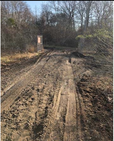
Photo 7. Access roadway to new monitoring wells after application of gravel and smoothing of ruts with Bobcat (TWS/ADT).
