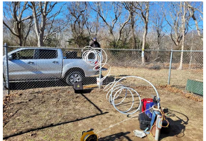
Photo 2. S76304 (Madison Hills Well 1) well redevelopment setup.
