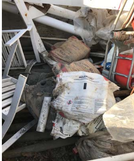
Photo 11. Materials disposed in Camp Hero Motor Pool dumpster by TWS/ADT; ADT will return to the site tomorrow (12/12/20) to remove the items from the dumpster to take back to their shop. (Photo by T. Dess.)
