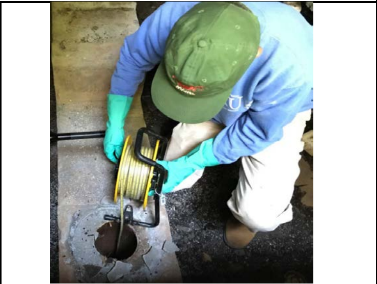
Photo 2. Supply well S17231 in pump house
