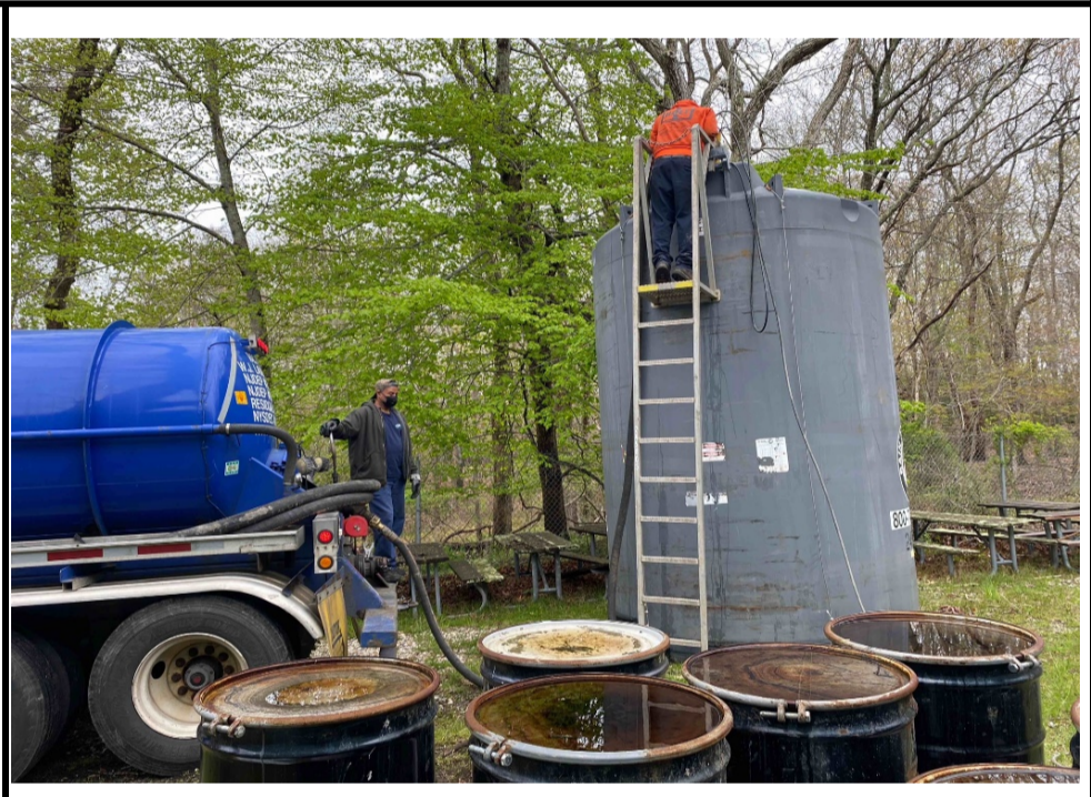
Photo 2. Liquid IDW being pumped out of frac tank.
