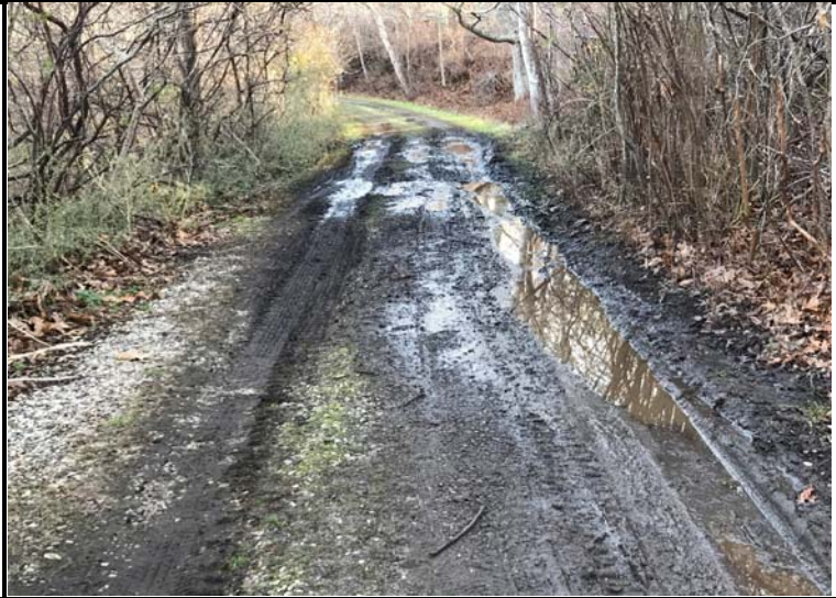
Photo 2. Ruts in the access path to Old Montauk Highway caused by vehicle traffic. USACE and AECOM will discuss restoration of the roadway with the State Park Superintendent.
