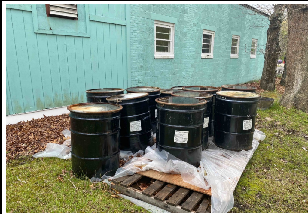
Photo 3. Soil IDW drum storage area at the motorpool prior to removal.
