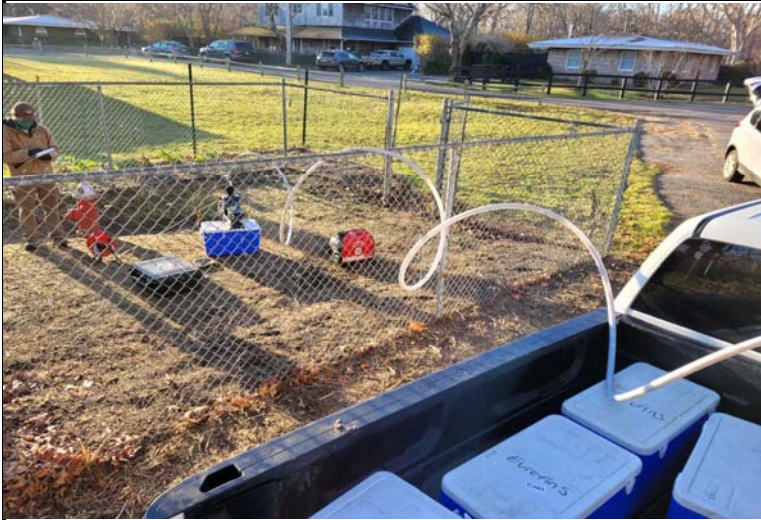
Photo 1. Well redevelopment at S 76304 (Madison Hill Well 1).
