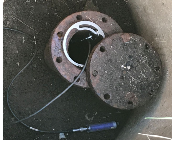
Photo 4. USGS active monitoring well along Route 27
