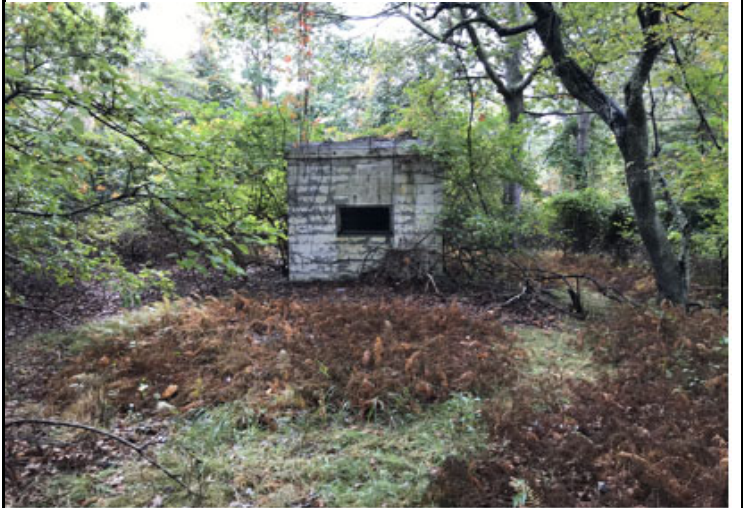
Photo 2. Former Supply Well S21084 pumphouse
