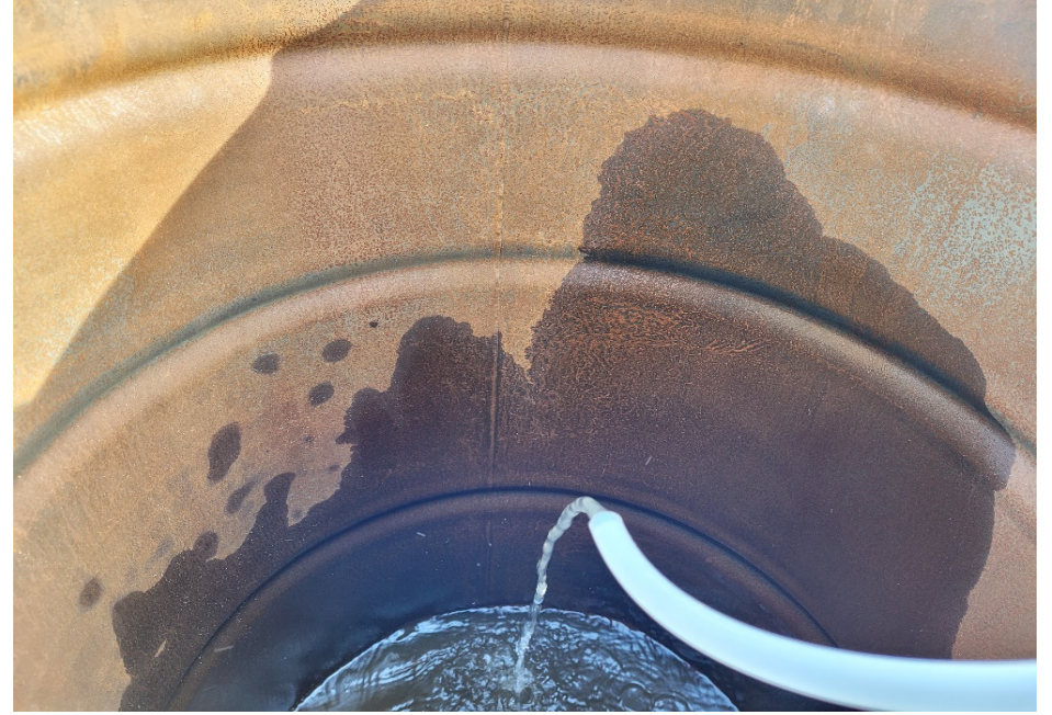
Photo 2. S76304 water quality; 84.2 NTU, steady 1 gpm discharge rate.
