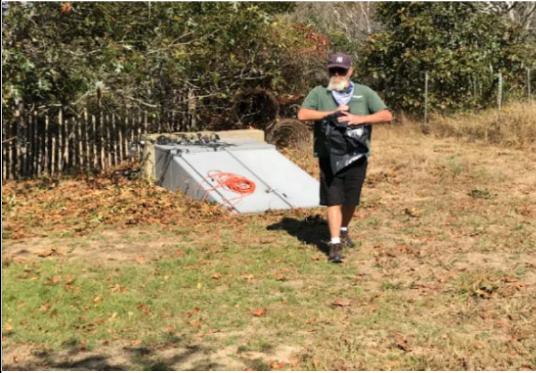
Photo 3. Montauk State Park well vault entrance
